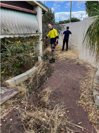
RESIDENTS FRONT GARDEN DURING THE RENOVATION PROCESS
